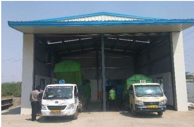
Compacting Machine Shed
